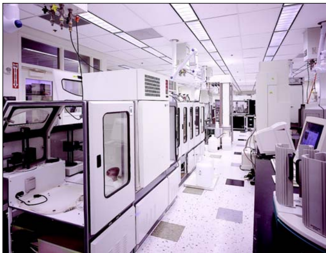
Figure 6. Service columns in areas of larger equipment.
