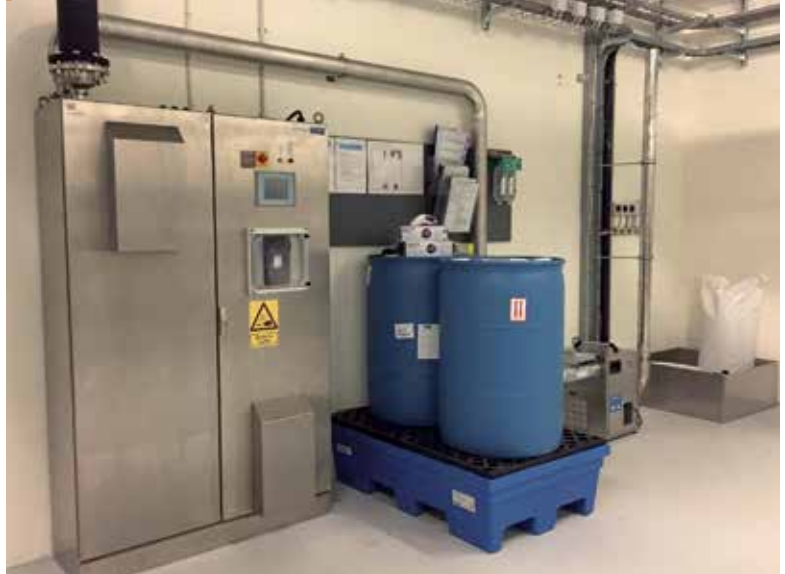
Figure 4: VPHP integrated generator with a continuous desiccant and bulk source of hydrogen peroxide solution
