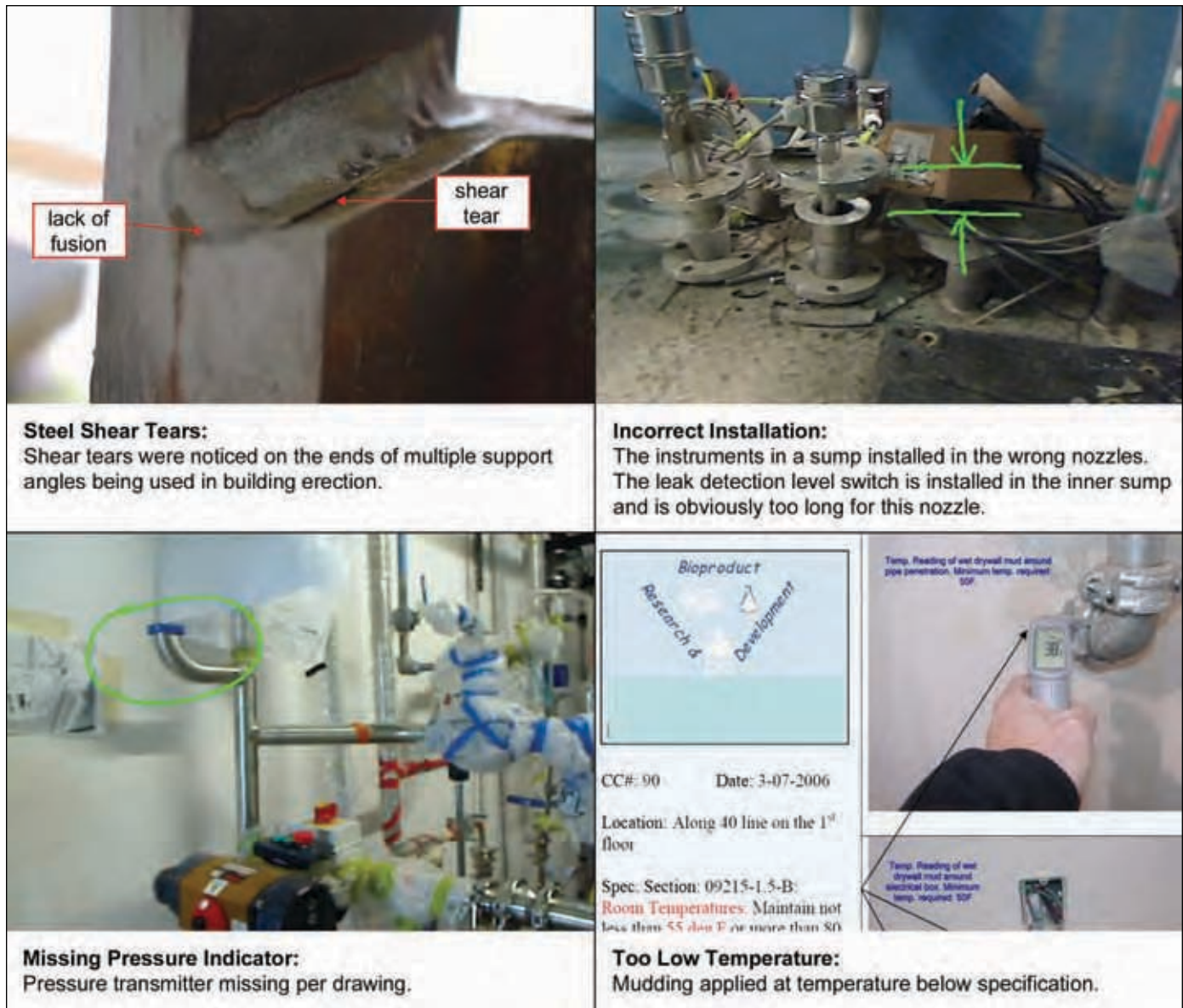
Figure 6. Typical construction quality related issues.
