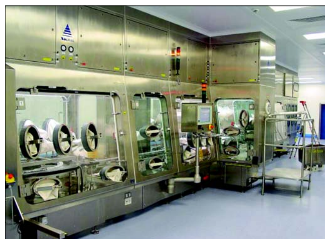
Figure 4. Isolated fill line, Aventis, UK. Photo courtesy SKAN AG.
